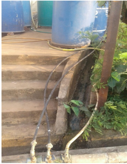
Figure 4.18 Running of Pipeline in slum
