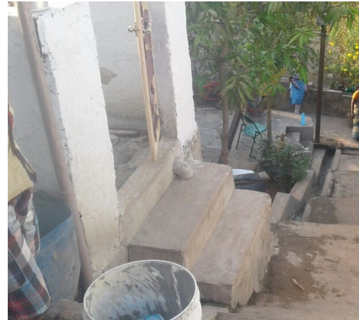
Figure 4.13 Location of storage tanks
